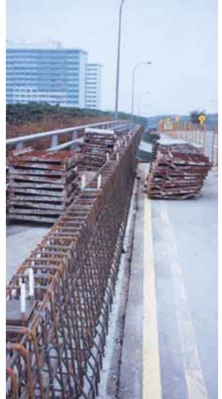
Parapet Wall Fixings
