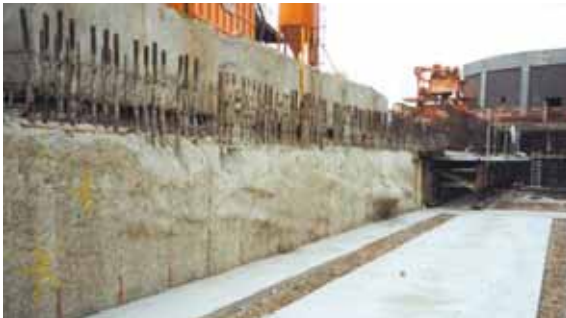
Diaphragm Wall Fixings
